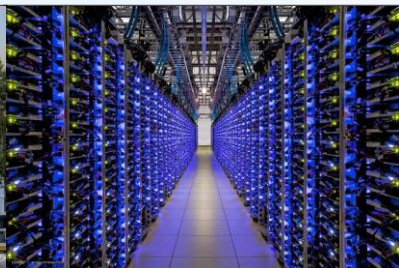
Bridge Data Center
