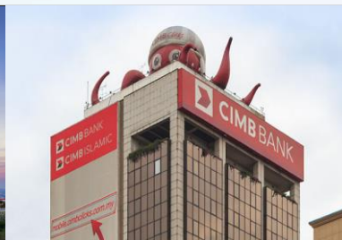
CIMB Bank, Putrajaya
